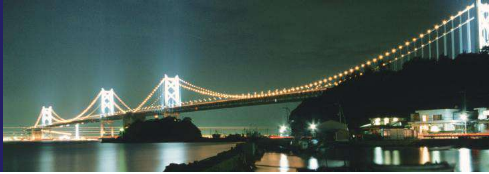
Photo provided by the Honshu-Shikoku Bridge Expressway Company Ltd. 照片由本州四國聯絡高速道路株式會社提供
